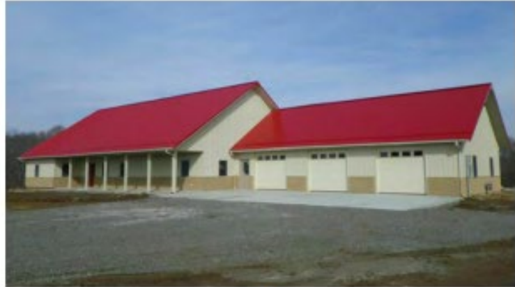
2 1 STORY METAL POST FRAME DWELLING W/ ATTACHED GARAGE
