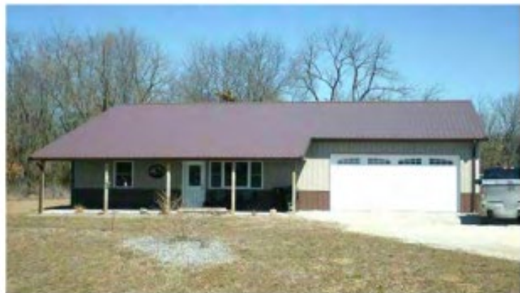
4 + 10 1 STORY METAL POST FRAME DWELLING W/ ATTACHED GARAGE
