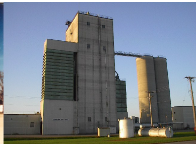
Good Concrete with Distribution Floor
