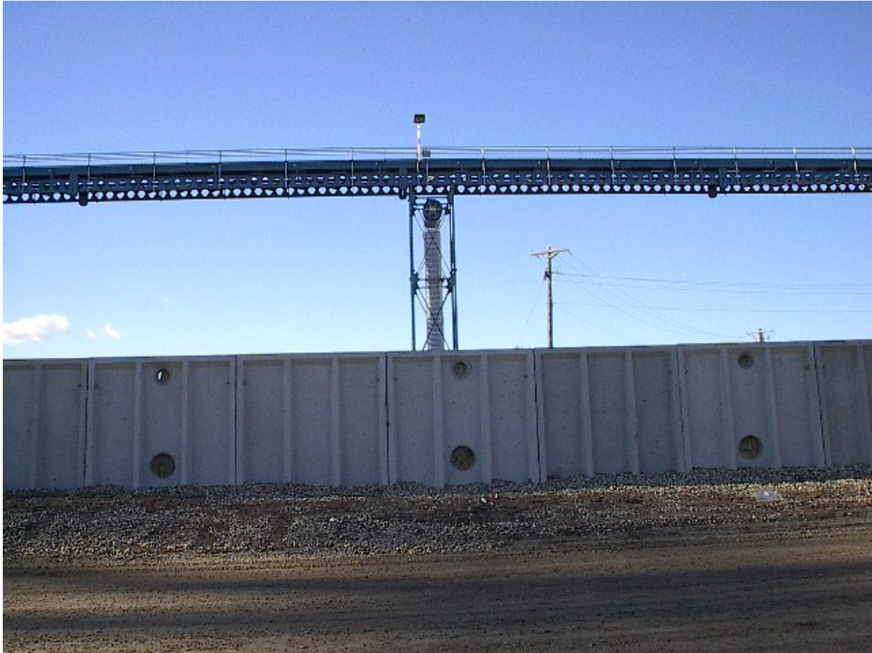
Concrete Sidewall Bunker
