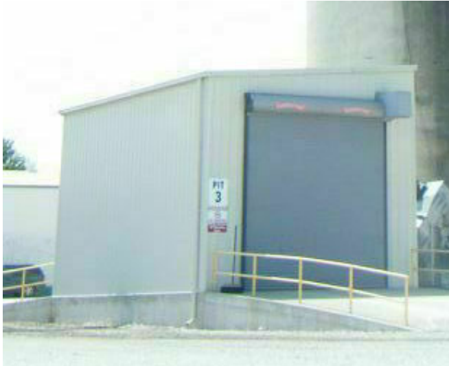
Enclosed Drive – Steel Frame
