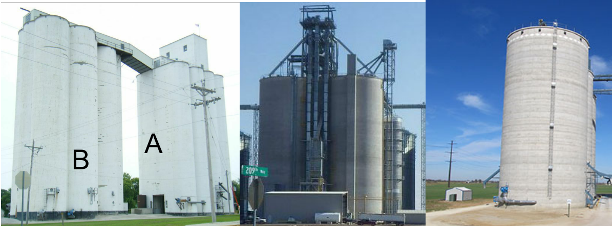
A. Average Quality Elevator with Head House B. Average Quality Annex with Intersticing Bins
